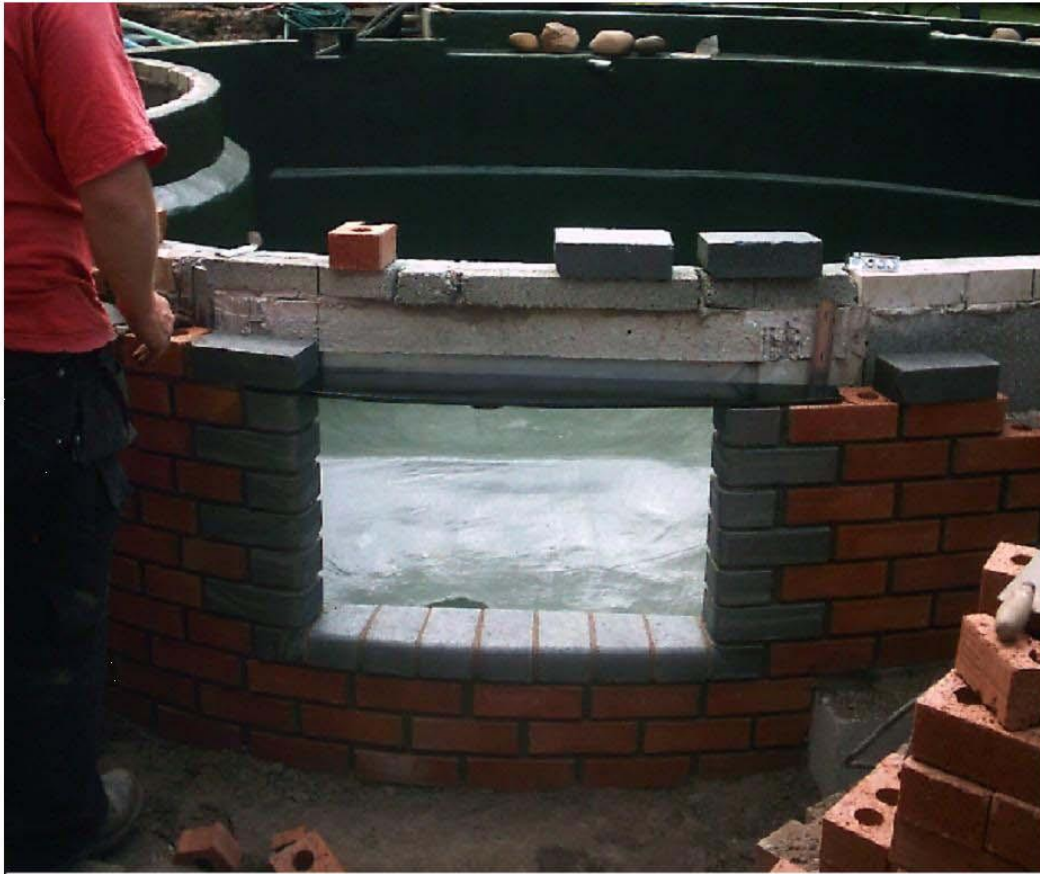
Ornate brickwork is laid to frame the viewing window. The outer skin of brickwork is added. Fibreglassing takes place.
