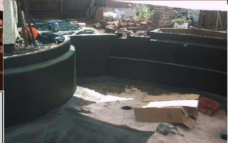
Ornate brickwork is laid to frame the viewing window. The outer skin of brickwork is added. Fibreglassing takes place.
