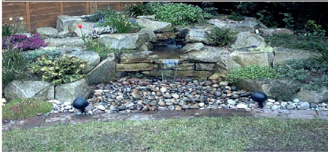
Feature Waterfall Using Butyl Liner and York stone. Cobbled area hides a sump of water housing the pump.
