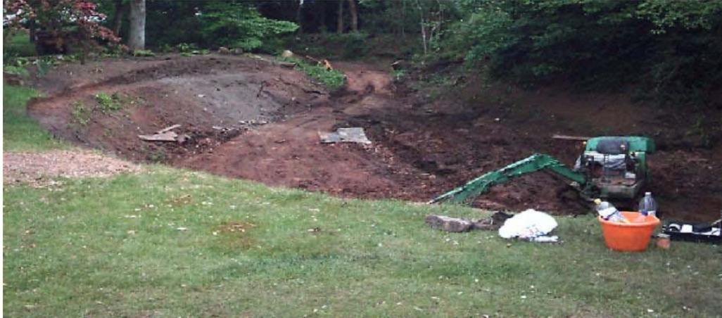
45000 Gallon Lake during the early stages of construction. The pool will be lined with Butyl Rubber.
